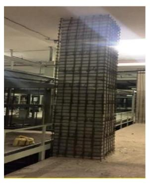
FIGURE 5: REINFORCEMENT CAGE AROUND THE EXISTING COLUMN, THE MAIN REINFORCEMENT IS ANCHORED INTO THE SLAB WITH CHEMICAL ANCHORING.
