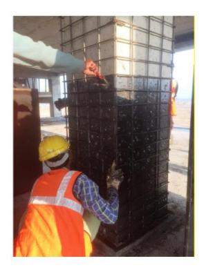
FIGURE 7: APPLICATION OF BONDING AGENT OVER THE EXISTING COLUMN.
