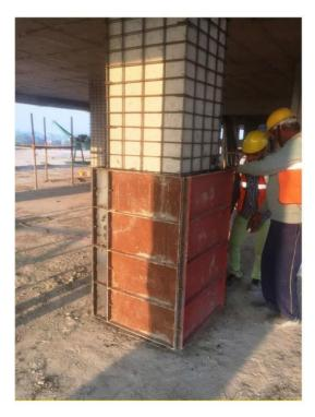
FIGURE 6: PROVIDING SHUTTERING AROUND THE COLUMN.
