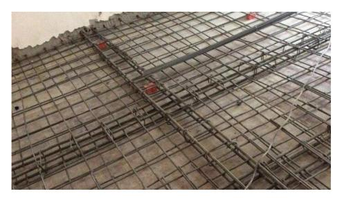
FIGURE 8: REINFORCEMENT MESH BOTTOM (OR TOP) OF THE FLOOR SLAB, THE MAIN REINFORCEMENT IS ANCHORED INTO THE BEAM WITH CHEMICAL ANCHORING.
